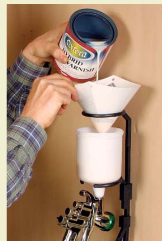
Filter the finish. Strain the finish through a cone filter to catch impurities that could clog the spray gun.
